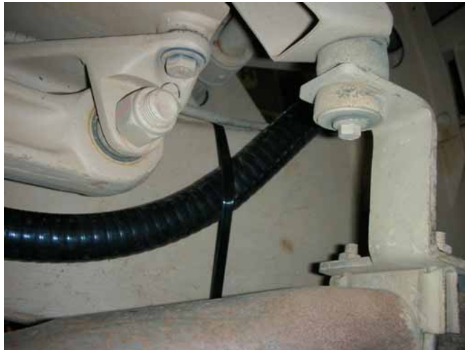
Figure 21 Securing the Conduit to the Chassis Rail
