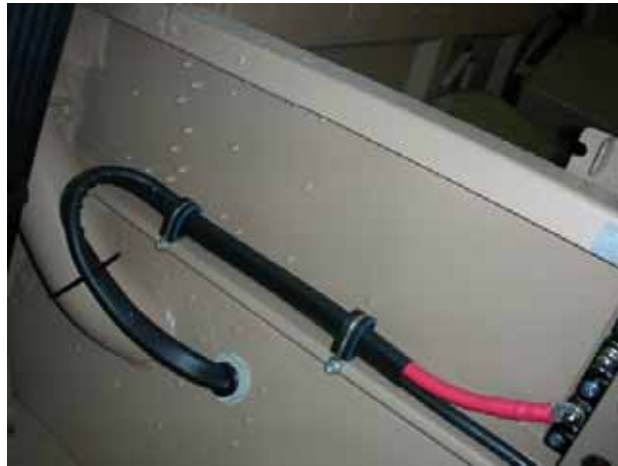
Figure 38 Routing and Securing of Load Centre Cables
