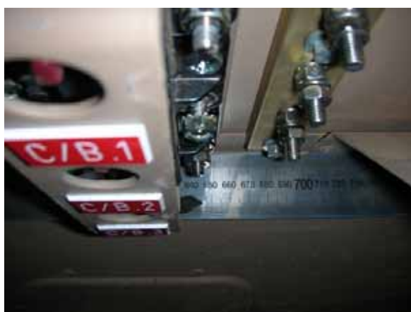
Figure 37 Installation of the Load Centre Earth Terminal Strip
